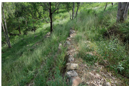
Fig. 1. A soil and water conservation structure for reforestation built through farmers' community work
