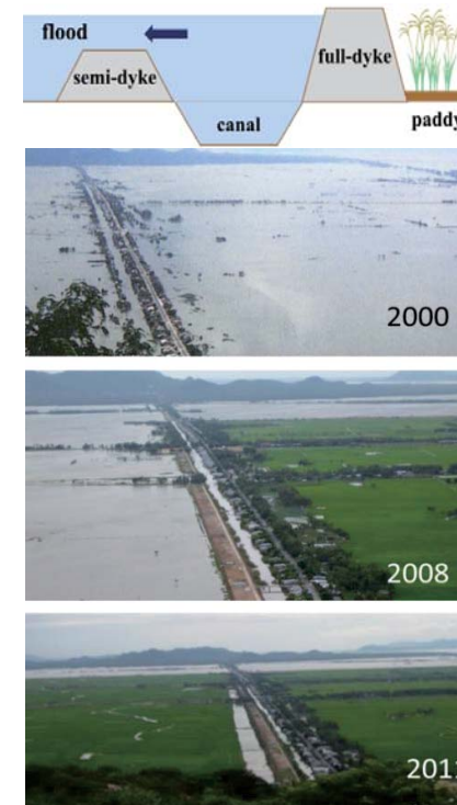
Fig.1 Semi-dyke and Full-dyke (Up: Both sides are semi-dyke area, Middle : Left; Semi-dyke area, Right: Full-dyke area Down : Both sides are full-dyke area)
