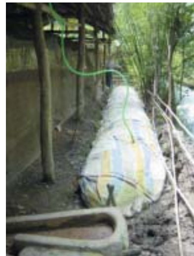
Fig. 2. Plastic biogas digester.
