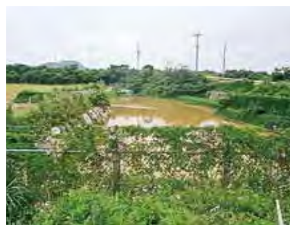
Sand basin installed in an upland field in Ishigaki Island
