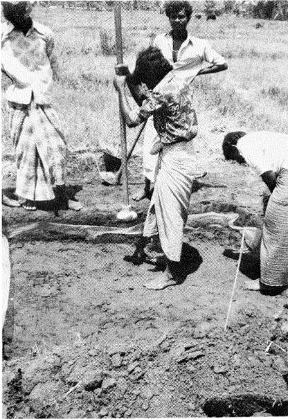
Photo.21 Preparation of a test plot for percolation control method (crushing and compaction)
