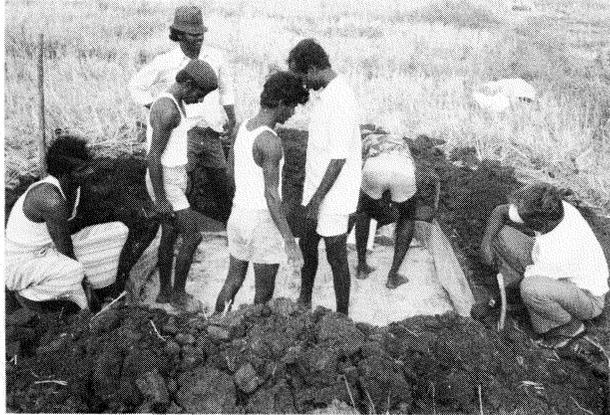
Photo.22 Preparation of a test plot for percolation control method (bentonite dressing (stratifying))
