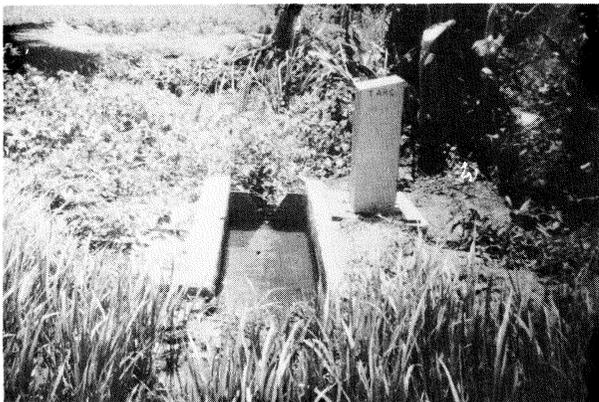
Photo.10 60° V-notch measuring wein installed at outlet of the detailed study lot.
