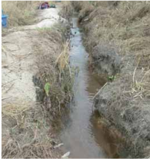
Figure 4-26 Damaged canal from water erosion
