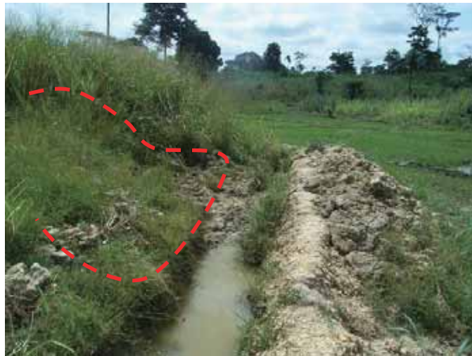
Figure 4-23 Damaged canal from landslide
