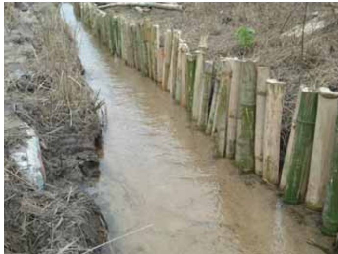
Figure 4-28 Bamboo Fence
