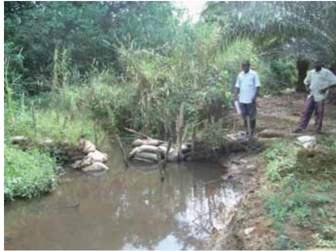
Figure 4-29 Damaged old dyke
