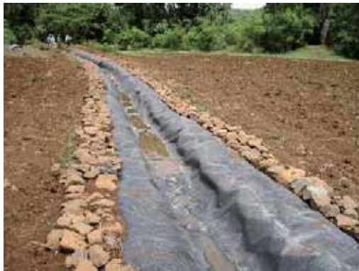
Figure 4-7 Canal covered with Geomembrane sheet (a) and Cross Section (b)
