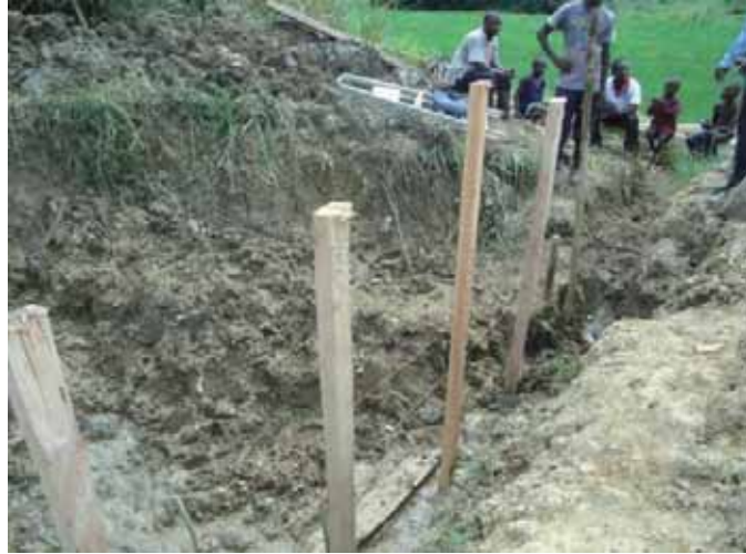
Figure 4-25 Pegging for Wooden fence
