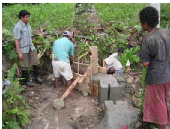
Aldeia inhabitants build the diversion gate under the guidance of JIRCAS and MAF officials
