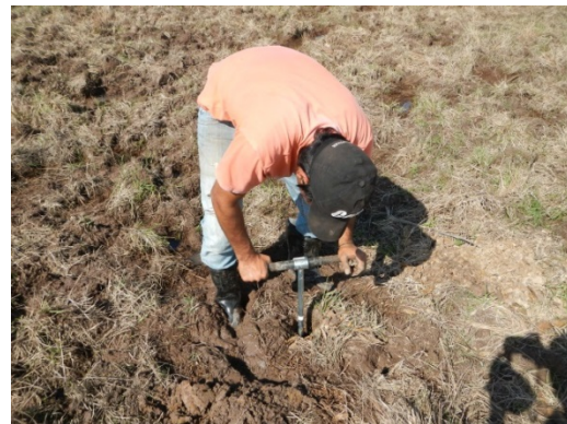
Reference Photo 2. State of excavation to install groundwater level pipes
