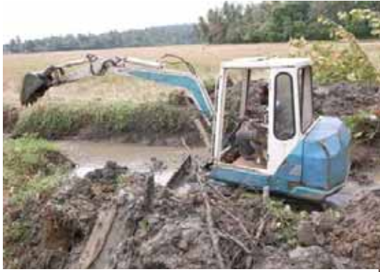
Pic.6.9 Hydraulic shovel working on the embankment
