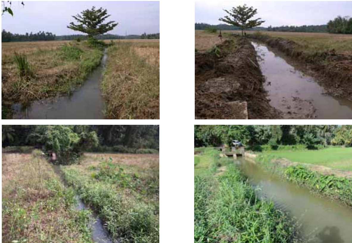
Pic. 6.8 Location where the flourishing weed and trees on the soil sedimentation could be an obstacle for the canal flow (before the works (left), and after the works (right))
