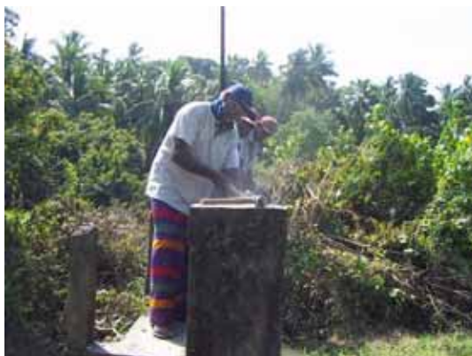
Pic.6.1 Removing the broken concrete body by using the hammer etc.
