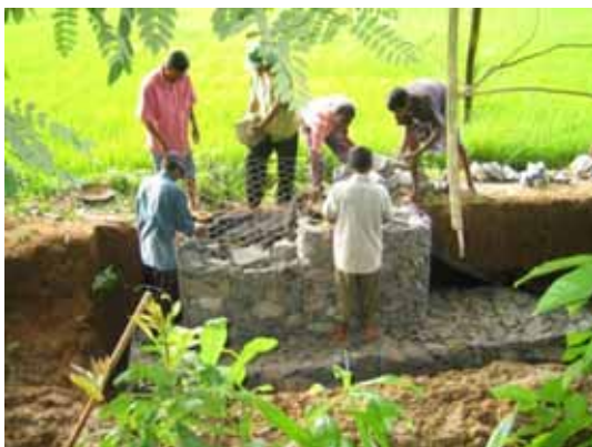
Pic. 6.13 Installation of the gabions
