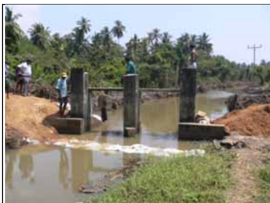
Pic.6.3 Sandbags stop water flowing to sluice gate rehabilitation section.
