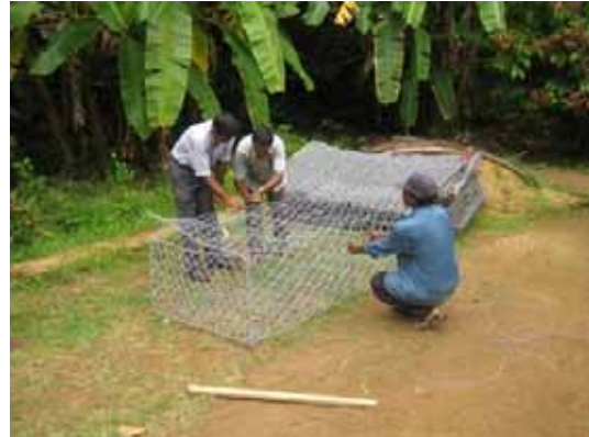
Pic.6.12 Building up the gabion
