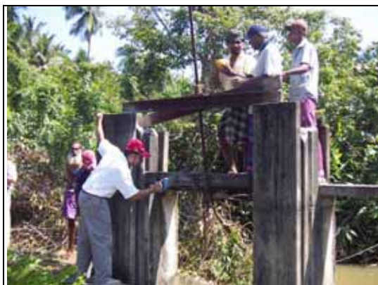
Pic.6.2 Removing the degraded wooden portion of the sluice gate
