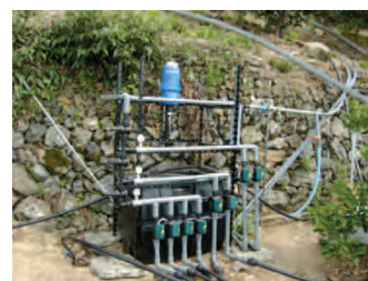
Figure 2 Drip fertigation system
