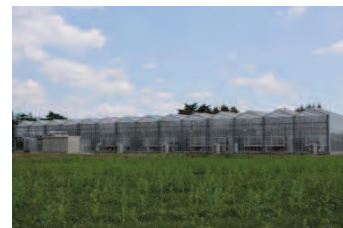
Figure 2 Plant factory in Tsukuba demonstration station installed with UECS
