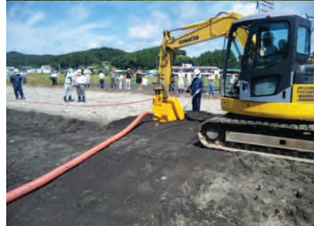
Scraping of the hardened topsoil
