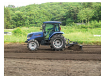
Scraping of topsoil by a tractor equipped with a rear blade
