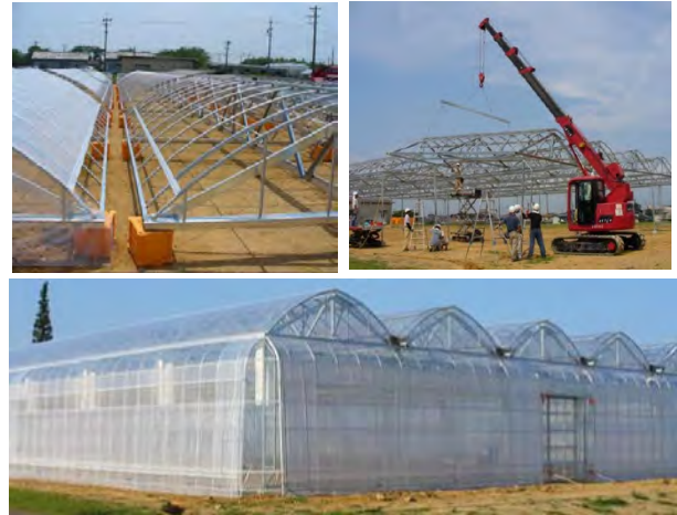
Figure 1 A very-low-cost and weather-resistant greenhouse built using unitized roofs
