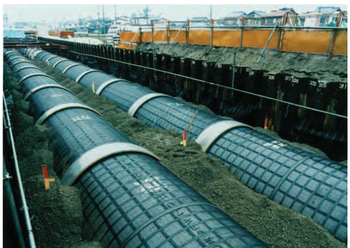
Laying of large-diameter pipelines using the shallow burying technique with geogrid
