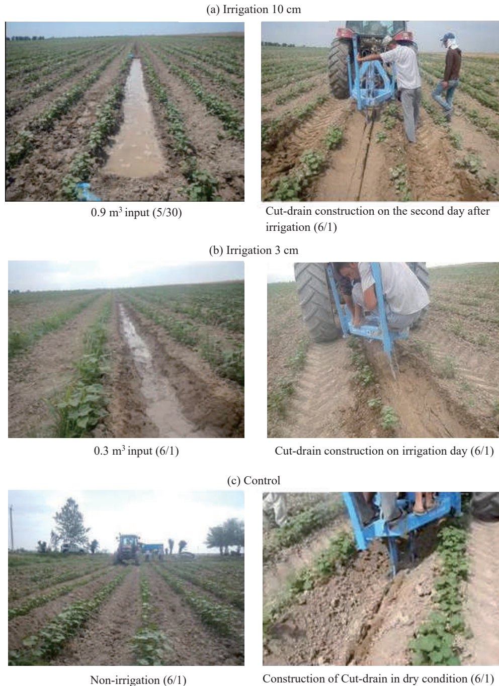
Fig. 6 Cut-drain construction under different irrigation conditions
