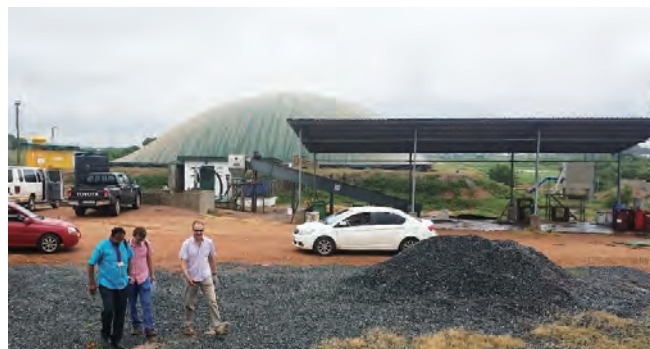
Safisana Biogas Plant in June 2017 (Tema, Ghana)
