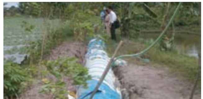
Photo2. Plastic type biogas digester set up by a farmer in Can Tho City ,Vietnam (Photo by E. Matsubara)
