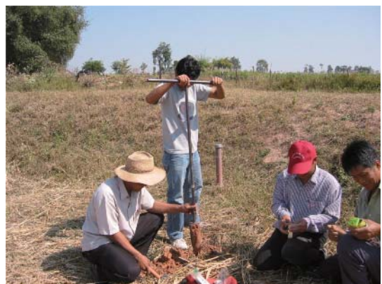
Photo 2. Lowland - Land use is for paddy fields during rainy season. Groundwater level was 0.5 m above the ground surface (depth of the well is 30 m) as measured on December 20, 2005.
