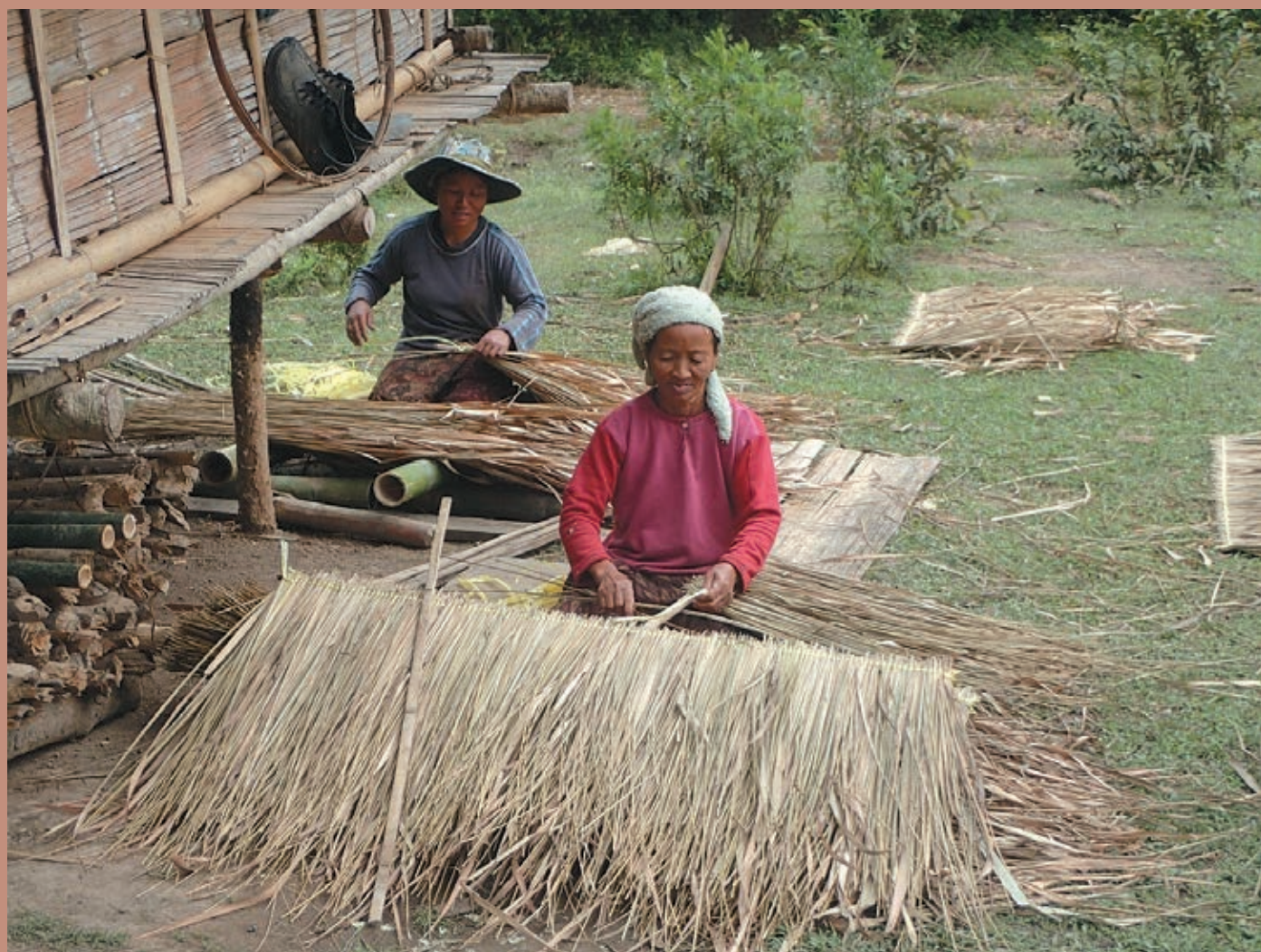
Building thatched roof panels with cogon grass in Laos (Photo by Dr. Hidetoshi Asai)
