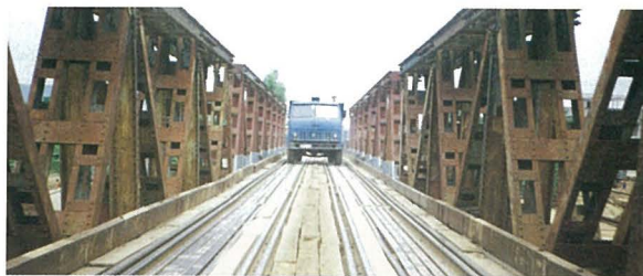
Photo 1: (Bridge): Trucks and trains run on the same bridge in National Highway No. 1
