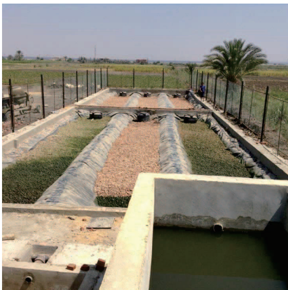
Fig. 6. Completed sewage treatment facility (View from the anaerobic tank to the stone and vegetation septic tank) Note: Photo by Embassy of Japan in Egypt
