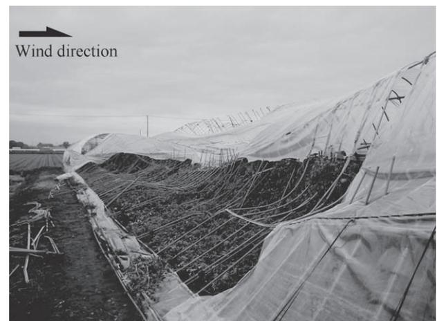
**Fig. 1. Collapse of a pipe house caused by strong typhoon winds (Moriyama et al., 2003)**
