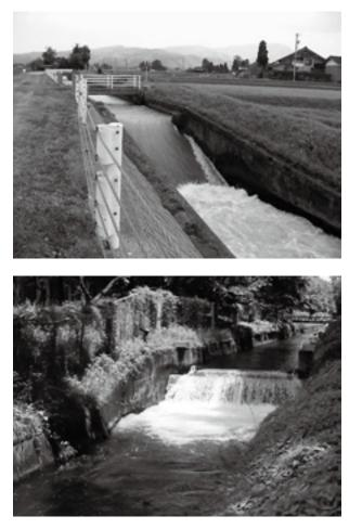
Fig. 2. Examples of a chute (top, Toyama Prefecture) and a drop (bottom, Tochigi Prefecture) along an irrigation channel
