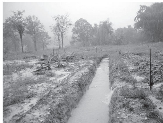
Fig. 10. Example of a small drainage ditch that has been dug near Bang Niang to enhance salt removal through drainage
