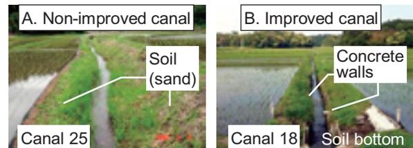
**Fig. 2. Non-improved drainage canal with soil walls (A) and improved drainage canal having concrete walls but with a soil bottom (B)**
