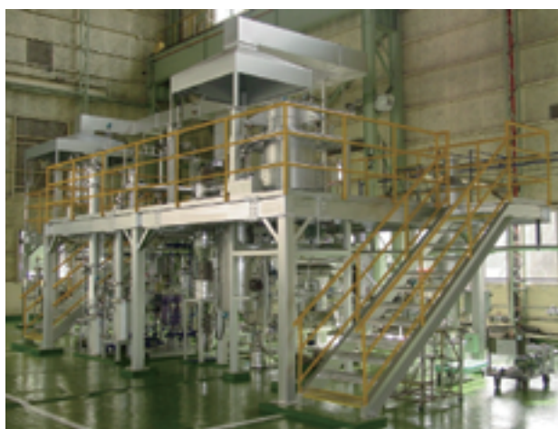
Fig. 7. “Norin Green No. 1”, a pilot plant of biomethanol production (MAFF and Mitsubishi Heavy Industries) Gasifier: 1) Capacity: 240 kg-biomass/day, 2) Type: entrained flow gasification, 3) Gasifying agent: oxygen and steam, 4) Pressure and temperature: normal pressure at 750–1,100°C. Methanol synthesis devise: 1) Capacity: equivalent to 20 kg-biomass/day, 2) Type: catalyst type, 3) Pressure and temperature: 30 kg/cm 2 g at 180–250°C.
