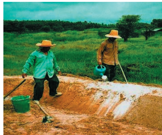
Fig. 6. Construction of water-impermeable dikes using a soil conditioner
