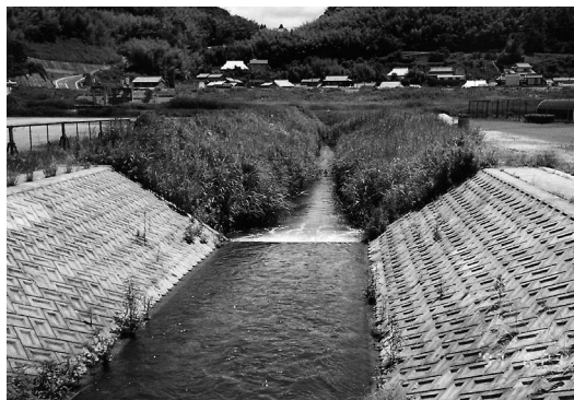
Fig. 5b. Drop directly below a sluice gate (Hata, June 1997)
