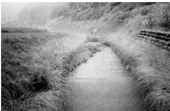
Fig. 4. Improved water channel in an upper watershed (Hata, July 1986) 1
