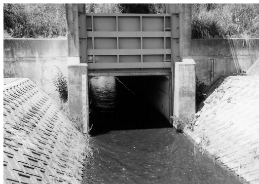
Fig. 5a. Discharge sluice gate on the Hyakken river (Hata, June 1997)
