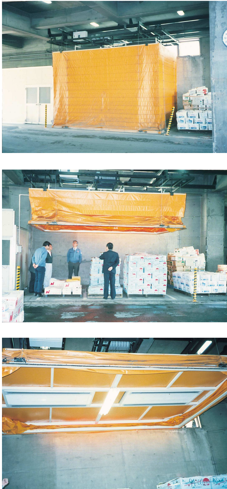
Fig. 2. Simple spotted cooling unit (SCU) 2
