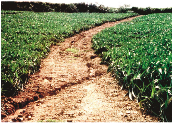
Fig. 1. A farm road in a pineapple field Rill erosion was observed along the farm road.
