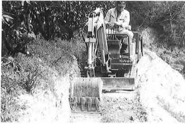
(1) Digging out using a small back hoe
