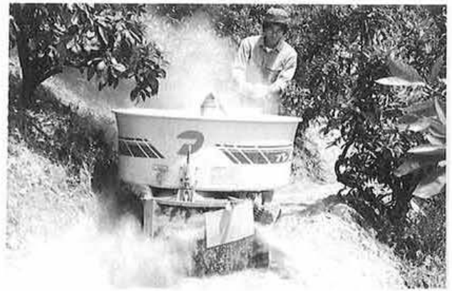
(2) Spreading cement and coagulant over the soil surface
