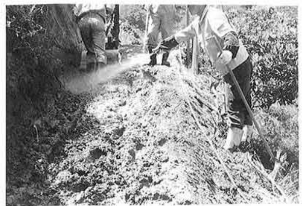
(4) Sprinkling water onto the mixture using a power sprayer
