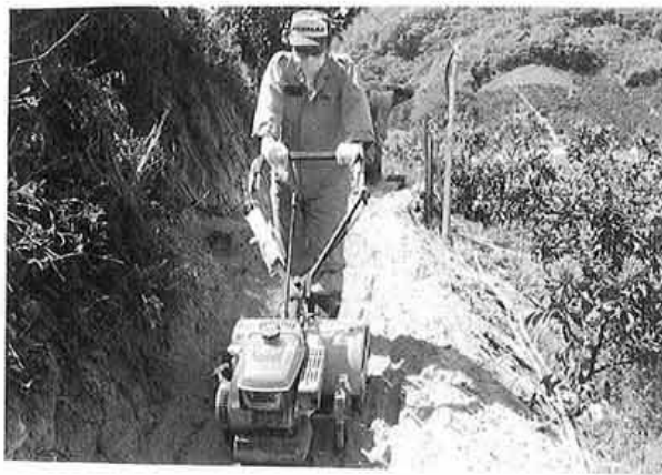
(3) Mixing together with soil using a rotary-tiller
