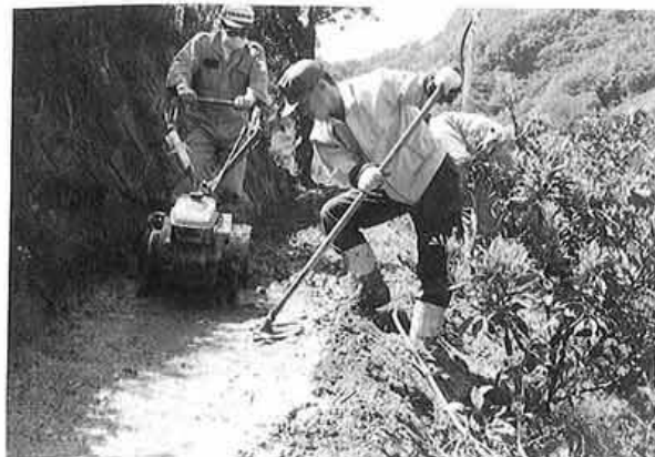
(5) Mixing all the ingredients and leveling out the surface
