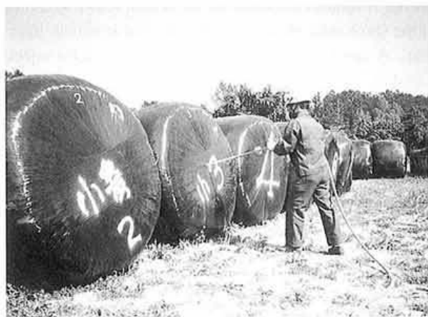
Fig. 2. Rapid and safe injection of ammonia
