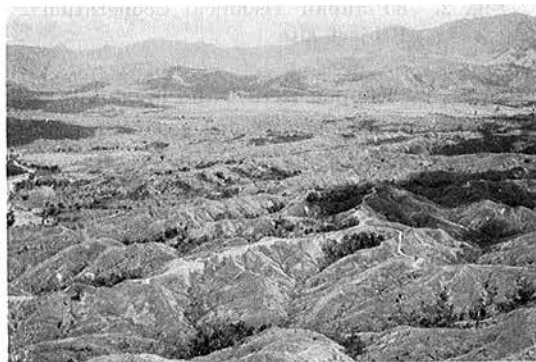
Plate 1. Project site (Parcel I and II)
