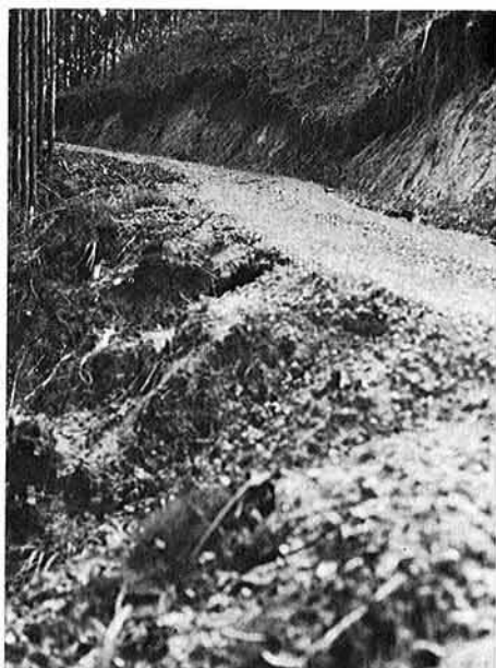
Plate 3. Feeder road through forest (gravel road)
