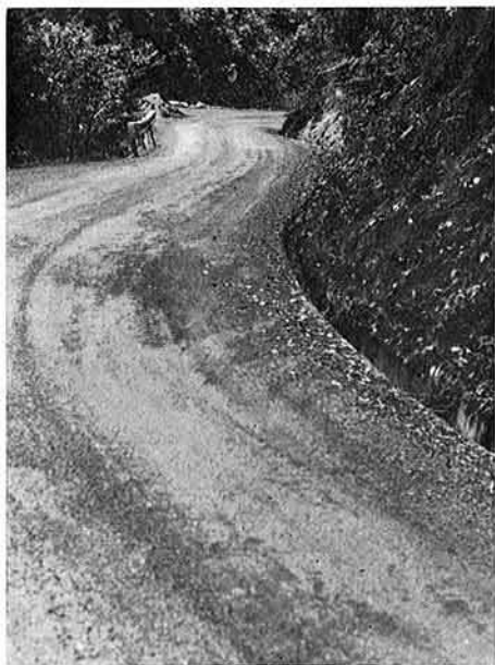
Plate 1. Multi-purpose trunk road (simplified pavement)
