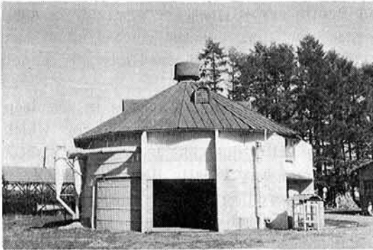
Fig. 4. Storage bin type drying shed in Tohoku National Agricultural Experiment Station
