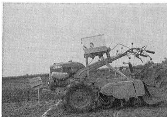
Fig. 1b Drill fertilizer with tillage attachments
