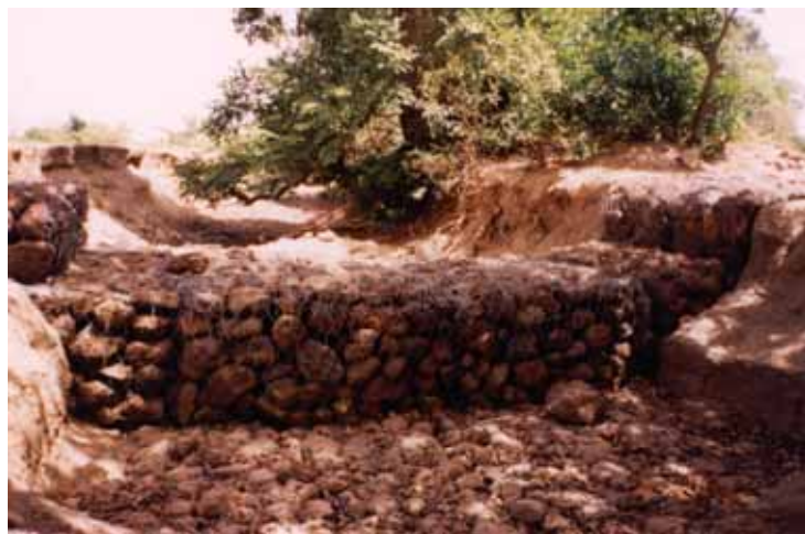
Figure 3.2.5.4 Example of large-scale restoration using gabion baskets
