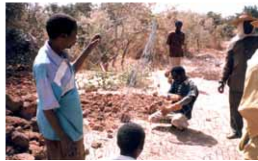
4. Assembling gabion baskets
