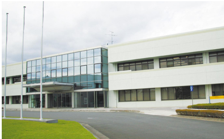
JIRCAS Main Building
