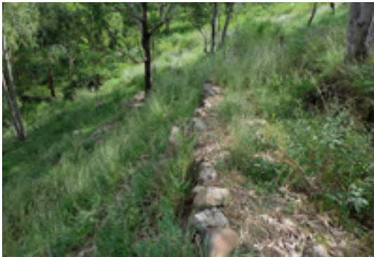
Fig. 1. A soil and water conservation structure for reforestation built through farmers' community work
