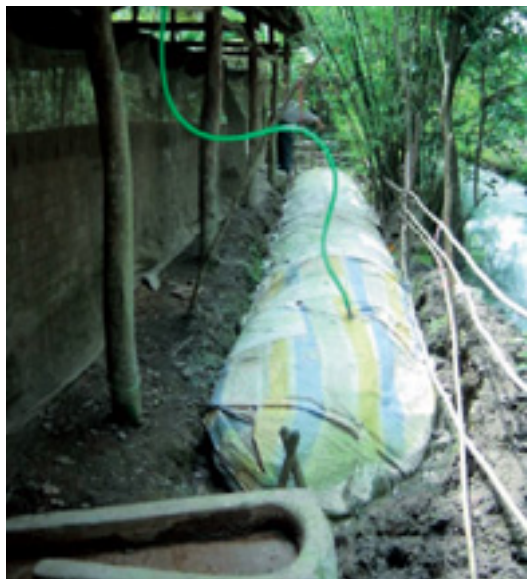
Fig. 2. Example of a biogas digester.
