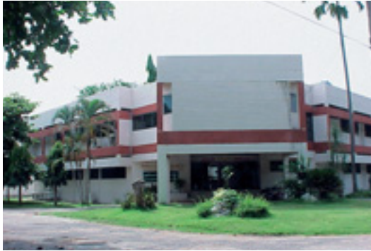
KKNRDC Main Building.
