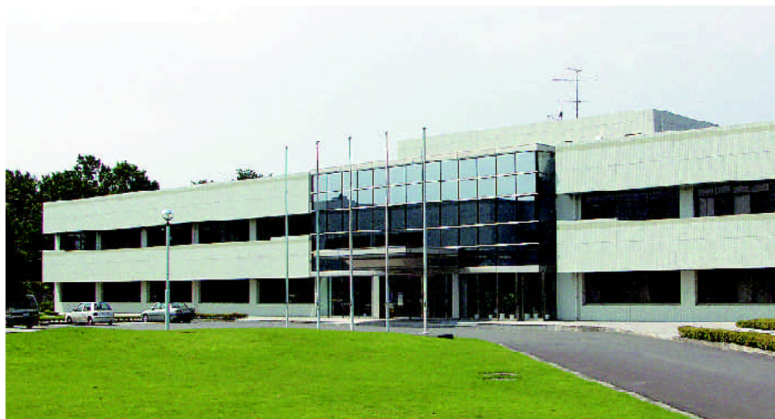
JIRCAS Main Building (Photo: T. Hayashi)
