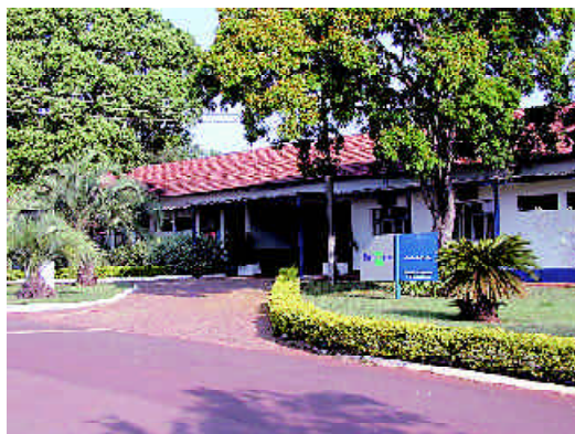
CNPGC's Main Building.
