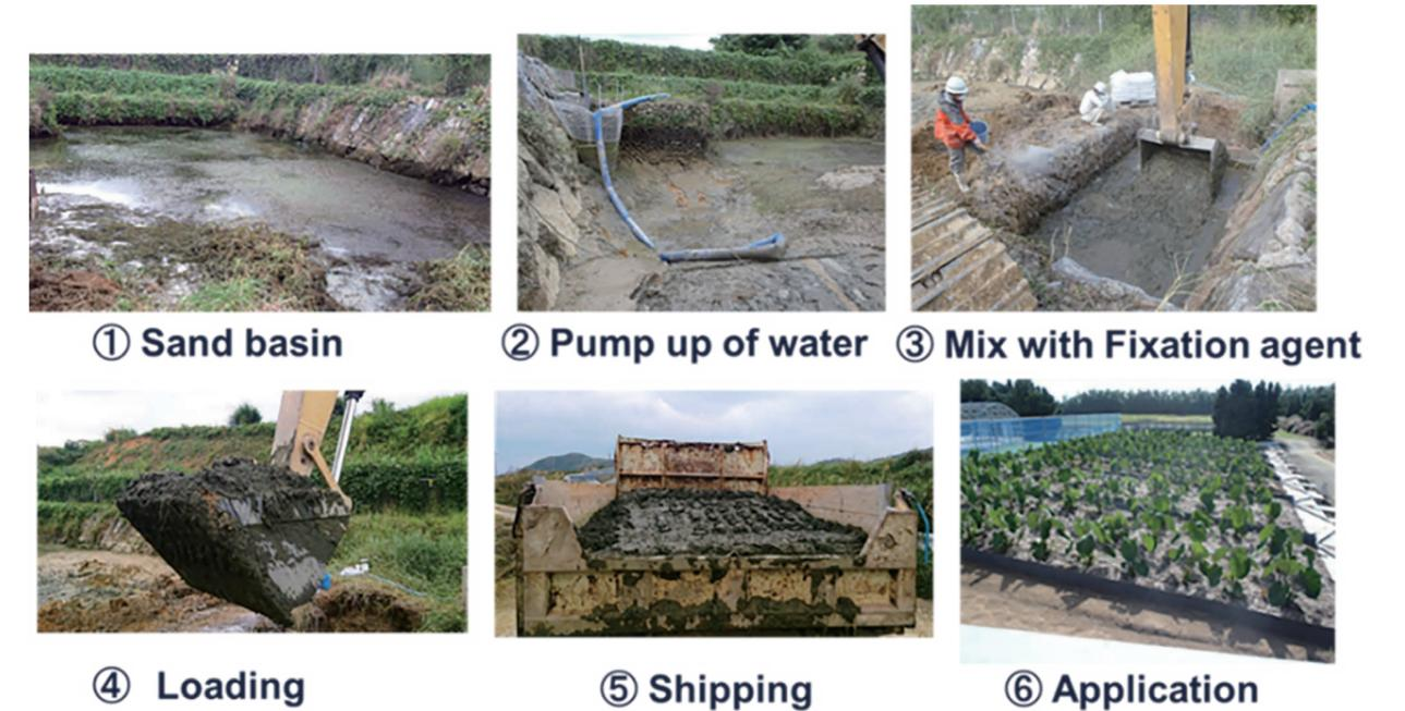
Fig. 46. Application of deposited soil in sand basin for taro production in Ishigaki
