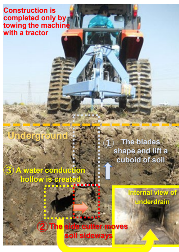
Fig. 3. How to create a water conduction hollow without pipes
