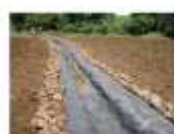
Figure 4-7 Canal covered with Geomembrane sheet (a) and Cross Section (b).
