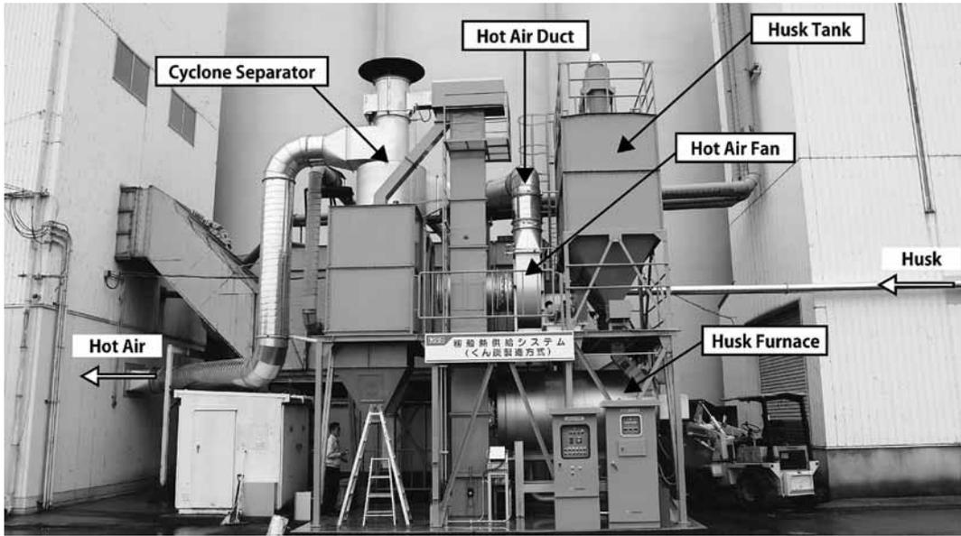
Fig. 2. Husk burner system
