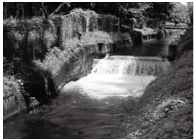
**Fig. 2. Examples of a chute (top, Toyama Prefecture) and a drop (bottom, Tochigi Prefecture) along an irrigation channel**
