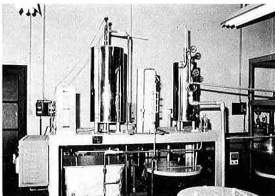
**Fig. 3. Continuous flow system pilot plant for chemical isomerization**
