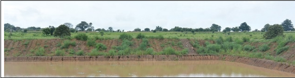
Inner slope covered with thatch material
