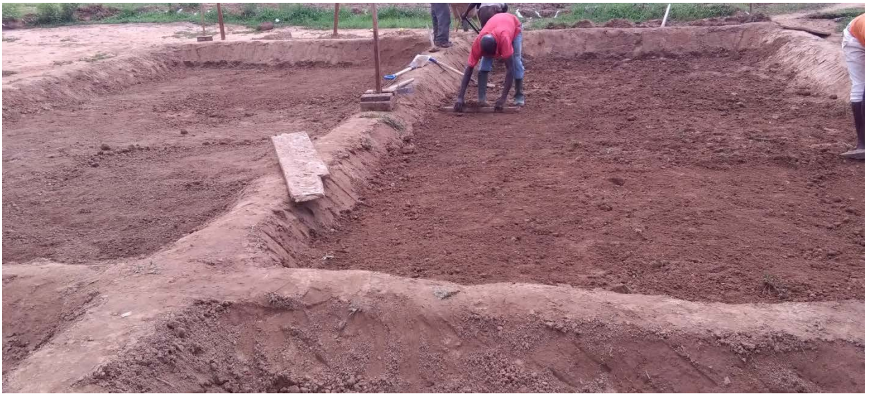
Fig. 2.41 Levelling of field inner perimeter
