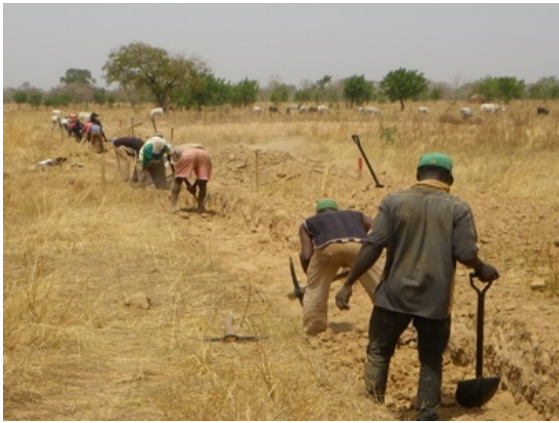
Fig. 2.13 Main canal construction
