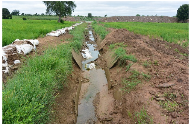
Fig. 2.12 Example of canal collapse
