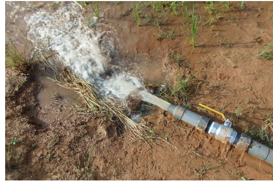
Fig. 4.3 A valve at the end of a pipe line
