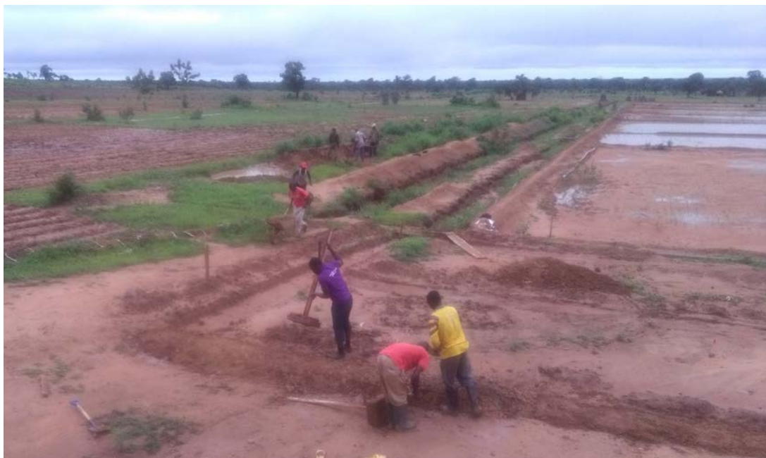
Fig.2.39 Bund compaction
