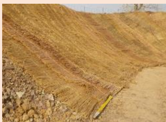
Fig. 2.24 Slope protection by thatch material
