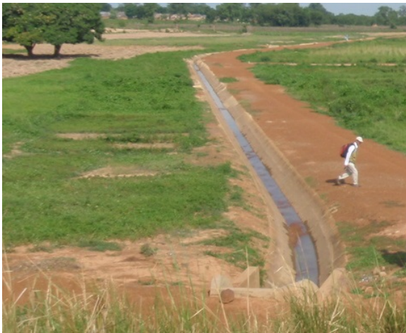
Fig. 2.15 Good example (the canal slope is gentle)
