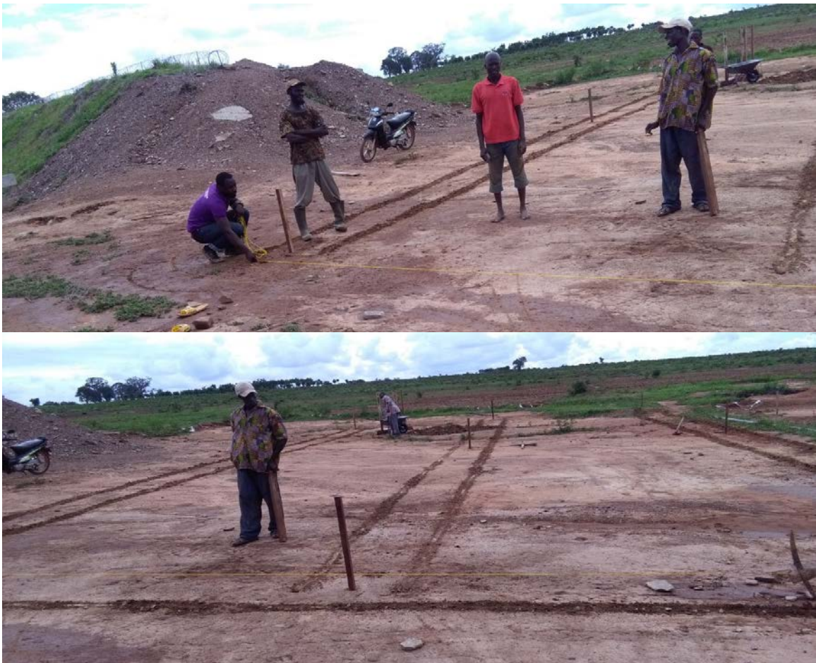
Fig. 2.36 Setting out field
