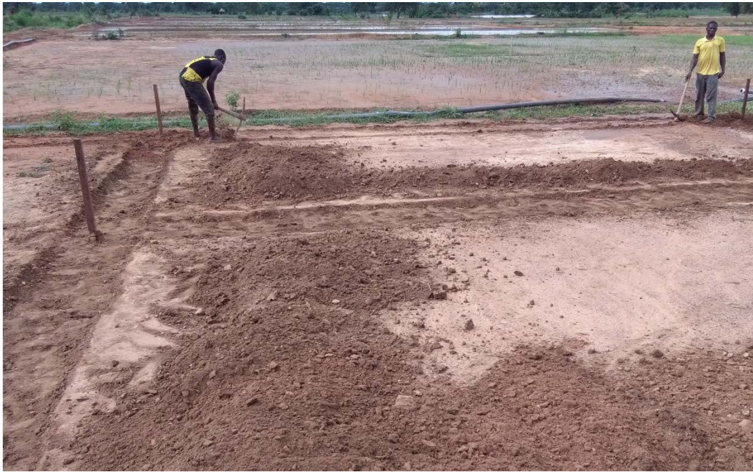
Fig. 2.38 Digging of trenches
