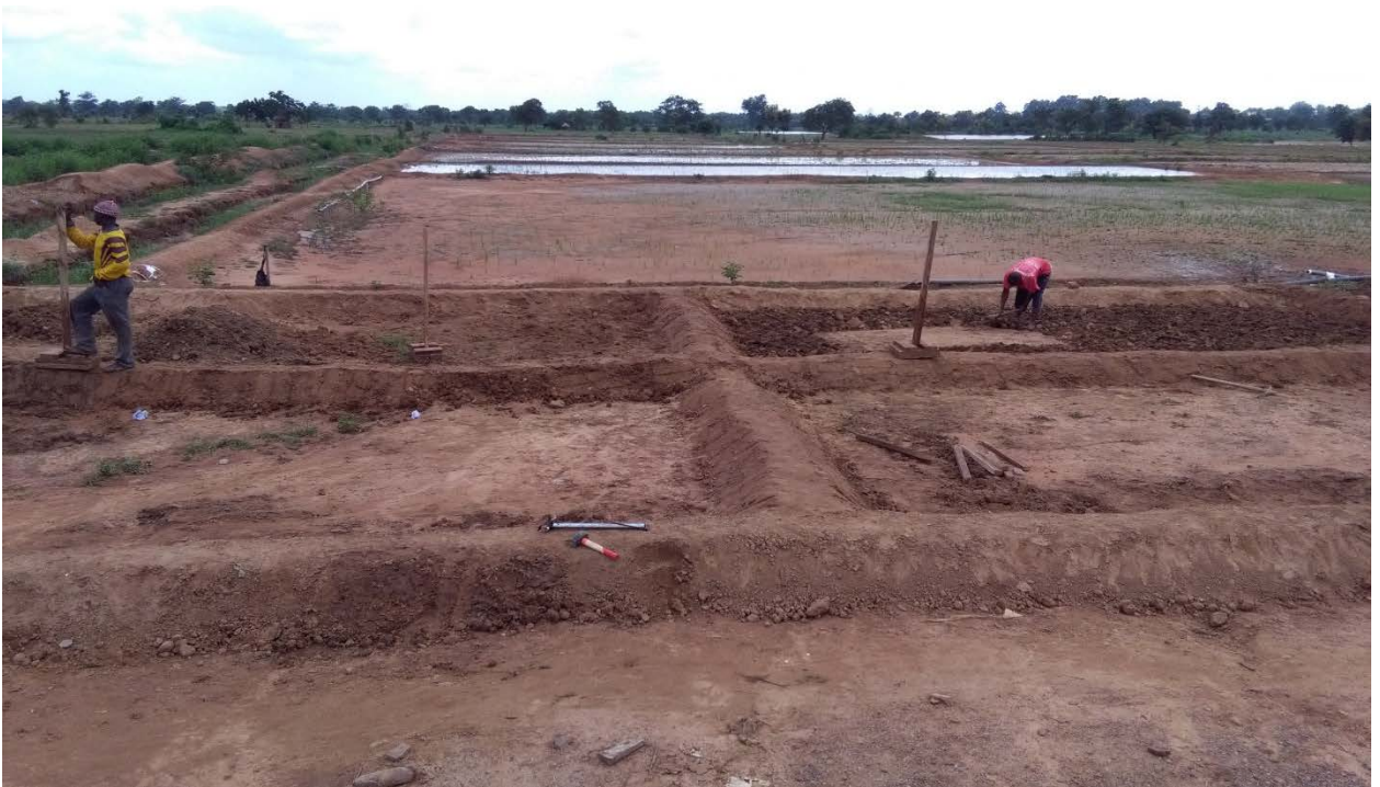
Fig. 2.40 Constructed bunds
