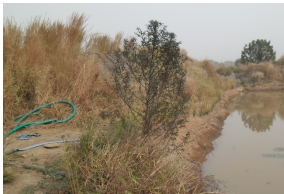
Fig. 4.11 Woody plant on the dyke of the sub-pond
