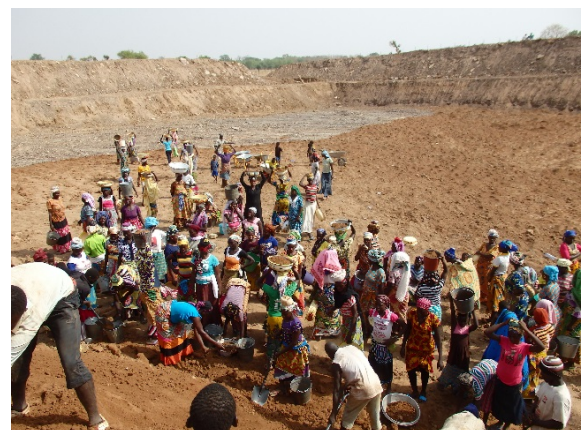
Fig.2.21 Mud laying in the sub-pond
