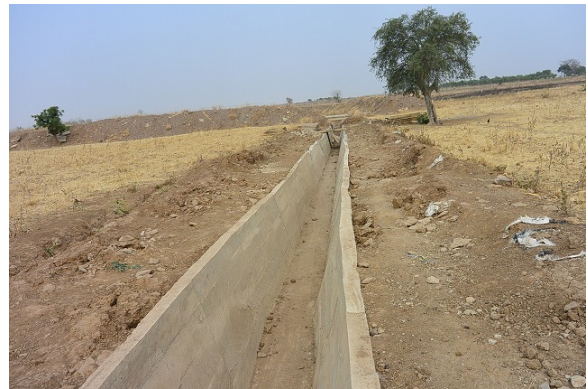
Fig. 2.14 Completed main canal (the canal slope is too steep)
