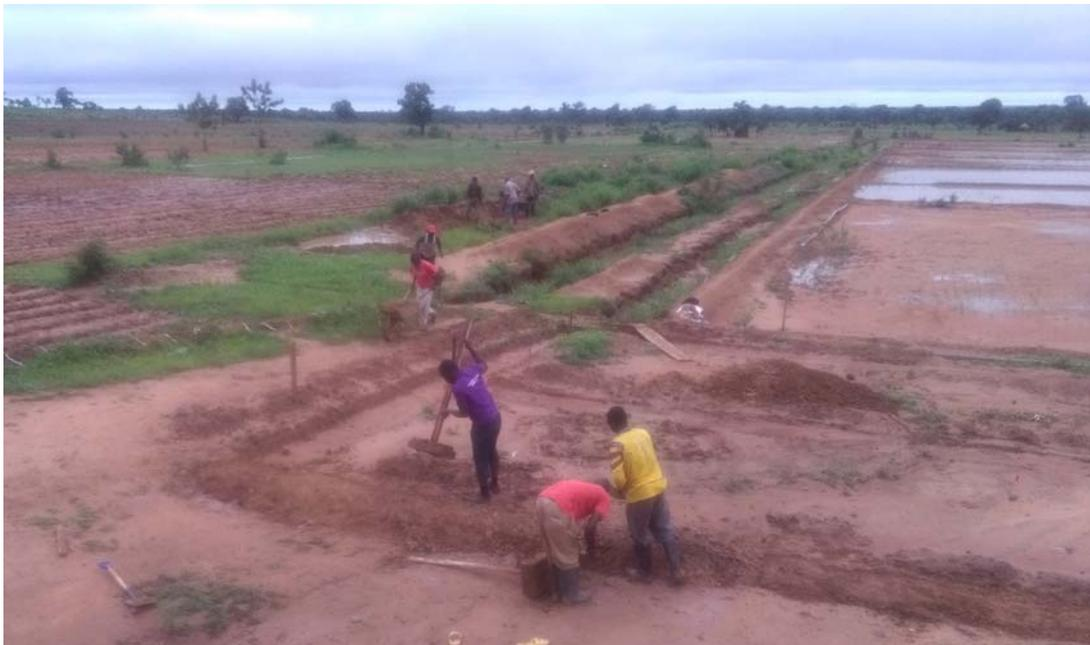
Fig.2.39 Bund compaction
