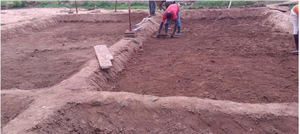
Fig. 2.41 Levelling of field inner perimeter
