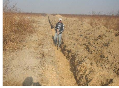
Installation of a hydrophobic material (Rice husk)
