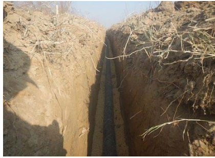
Lateral drain in a shallow sub-surface drain
