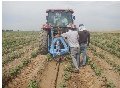
Construction of auxiliary drains (cut-drains)
