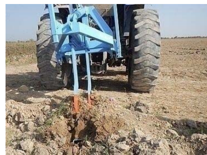
Fig. 4.3.12 Uplifting the drilling unit
