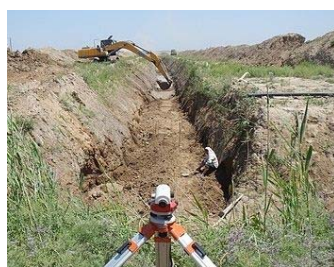
Cross-section of deep sub-surface drain
