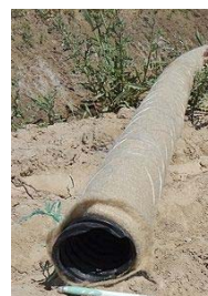
Lateral drain to be installed
