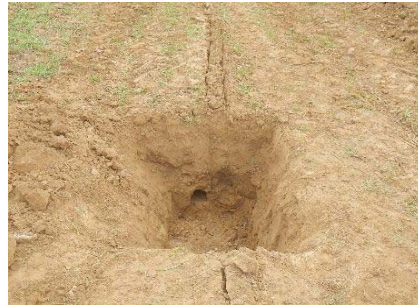
Hollow of a cut-drain
