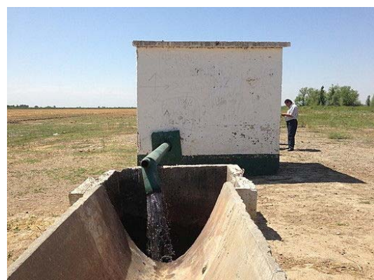
Fig. 2.1.12 Vertical drainage facility
