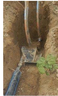
Dragging starts at the soil cross-section (The thicker pipe at the front is a guide pipe.)
