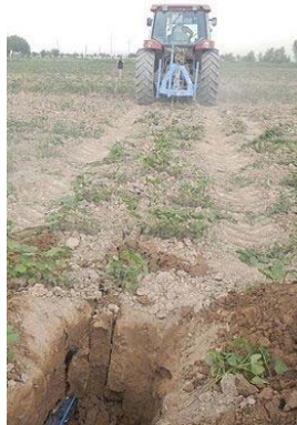
Dragging of a pipe
