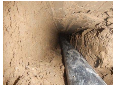
A pipe drawn into the hollow (diameter 50 mm)
