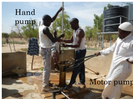
Photo 6.4.2 Installing pumps
