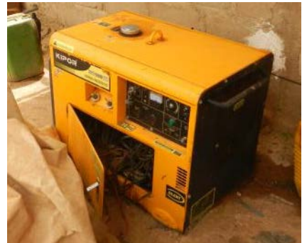
Photo 6.7.2 Diesel Power generation
