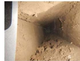
Cut-drain hole after construction
