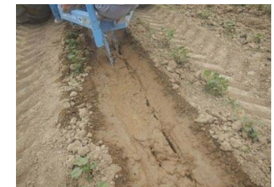
Construction of a cut-drain immediately after irrigation
