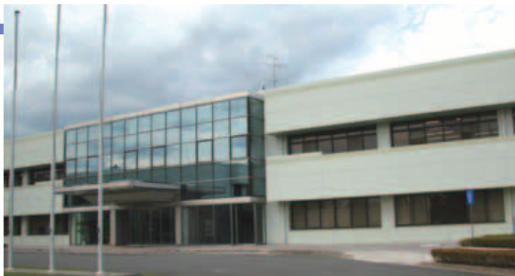
JIRCAS Main Building.
