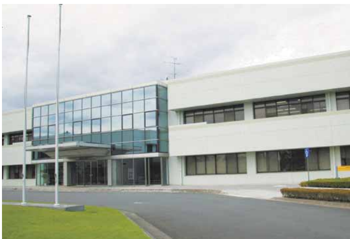
JIRCAS Main Building.
